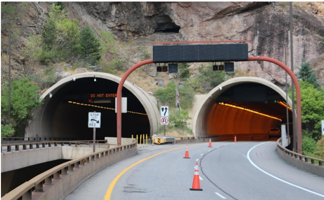
Figure 24. View of east portals for the Hanging Lake Tunnels, view facing west. Mead & Hunt, Inc. photograph.
