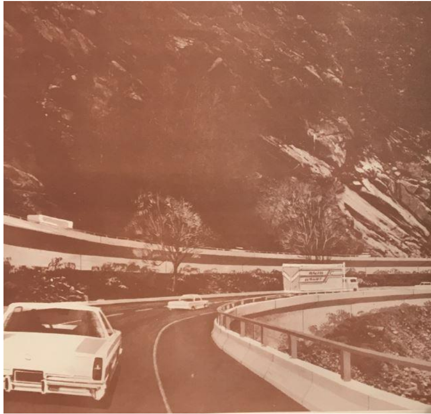
Figure 22. 1979 rendering of terraced roadway with retaining walls and landscaping. Note the shadow cast on the retaining wall by the cantilevered roadway; this was an aesthetic choice to soften the visual impact of the retaining wall. 122
