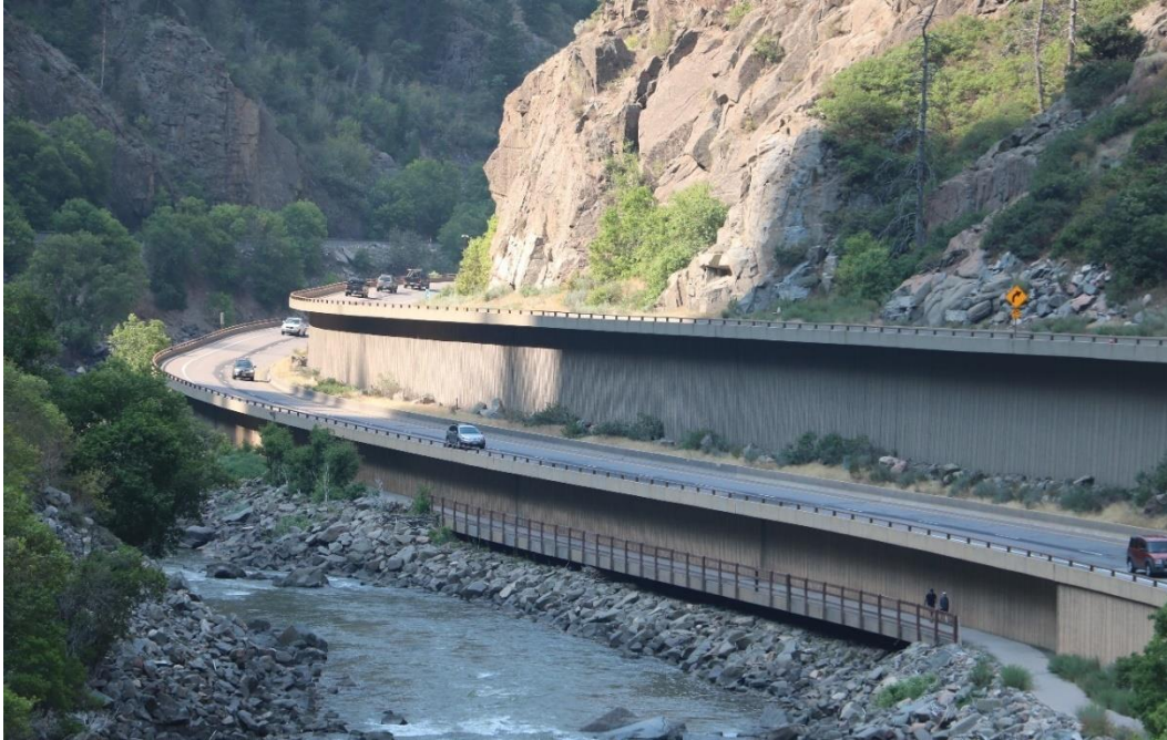
Figure 23. View showing terraced roadway, retaining wall, and cantilevered overhang with shadow. Note the location of the recreational path below the cantilevered eastbound travel lanes. Mead & Hunt, Inc. photograph.
