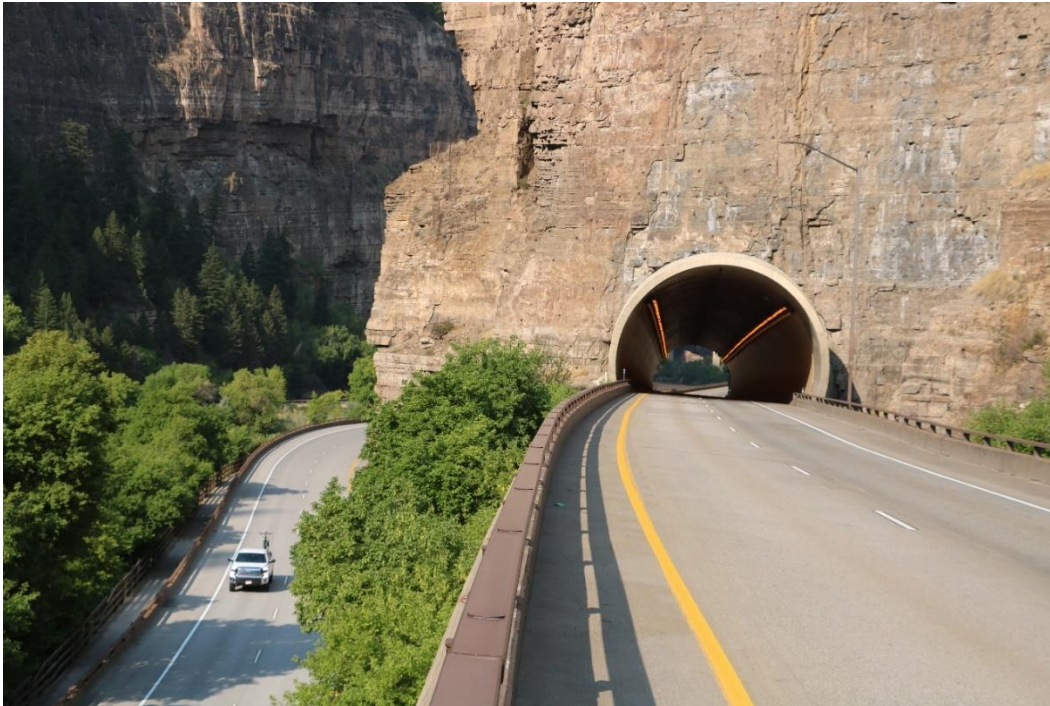
Figure 26. View of Reverse Curve Tunnel with eastbound roadway below, view facing west. Mead & Hunt, Inc. photograph.
