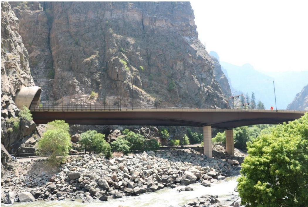
Figure 16. Welded steel girders on at the west portal of the Hanging Lake tunnels featured variable depth girders. Mead & Hunt, Inc. photograph.
