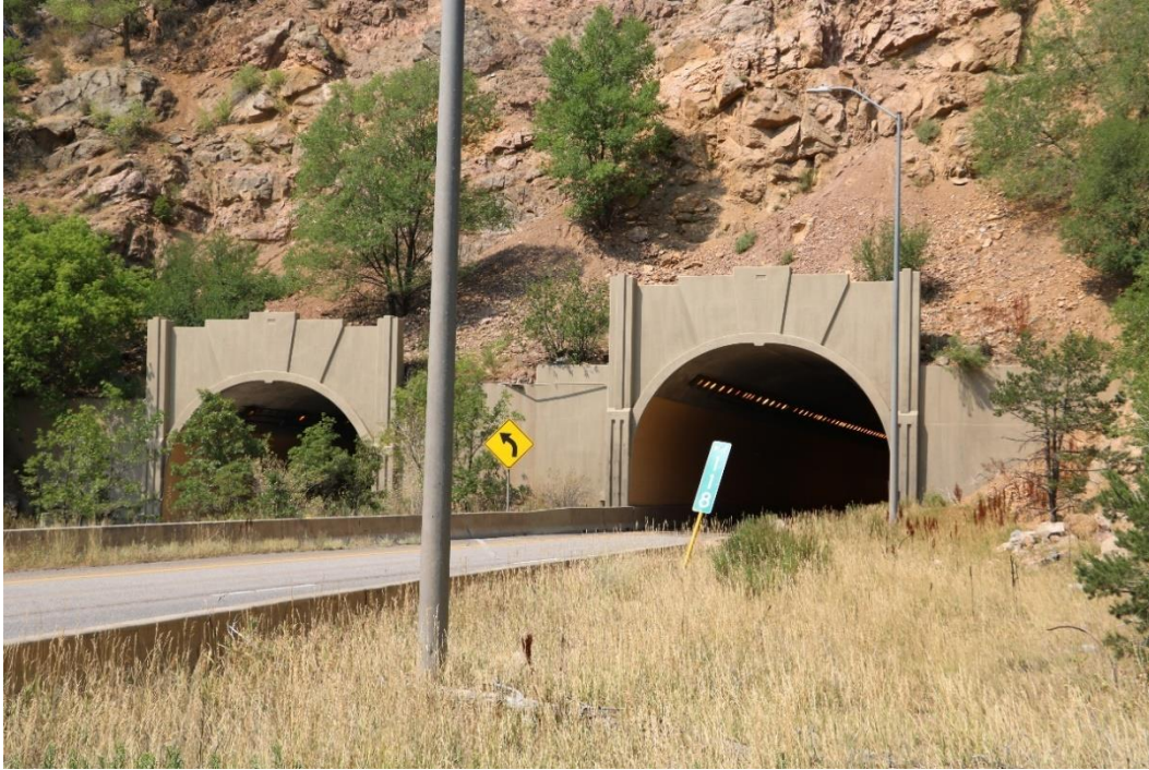
Figure 2. The twin tunnels located west of No Name were completed in 1965. Mead & Hunt, Inc. photograph.
